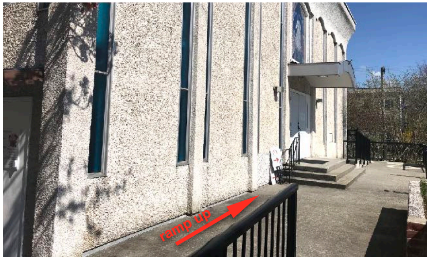
Photo showing the last section of the 'accessibility ramp' arriving at the entrance podium but more stairs at the church entrance doors are left to tackle.
