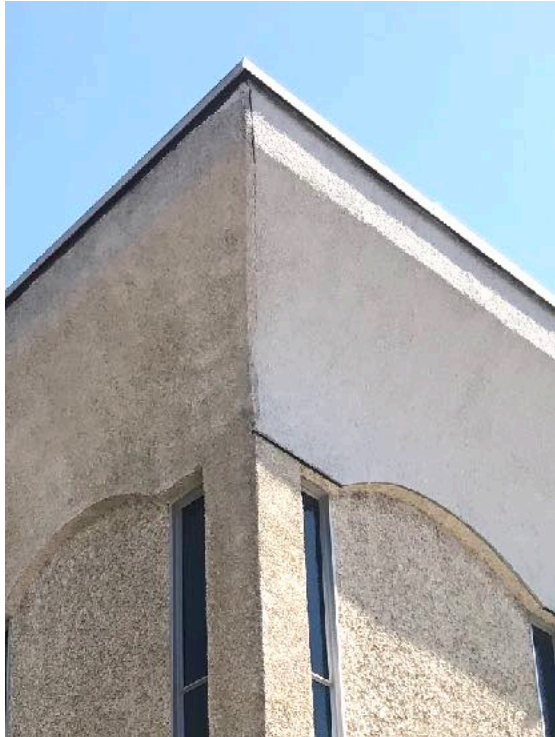
Above left: Cornice at corner of parking lot and lane showing a crack in the stucco.
