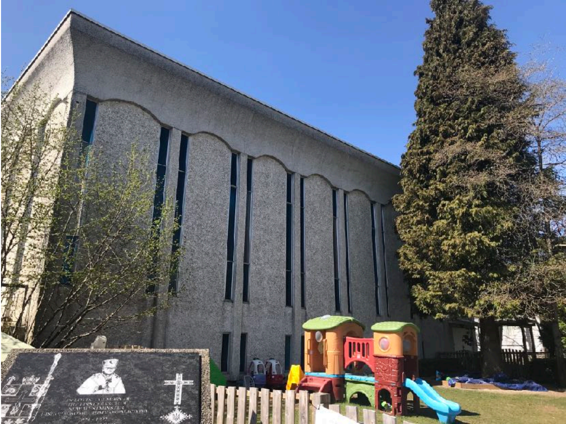
Side view (facing 5th Street)
