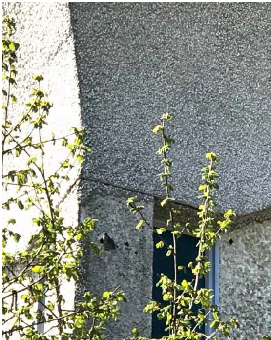
Above right: Cornice at corner of lane and yard showing missing/failing stucco just below an new roof drain installed 13 years ago. Below left: Cornice at corner of front and yard showing stucco damage caused by woodpeckers below Right: Evidence of moisture staining on stucco below windows at parking lot.
